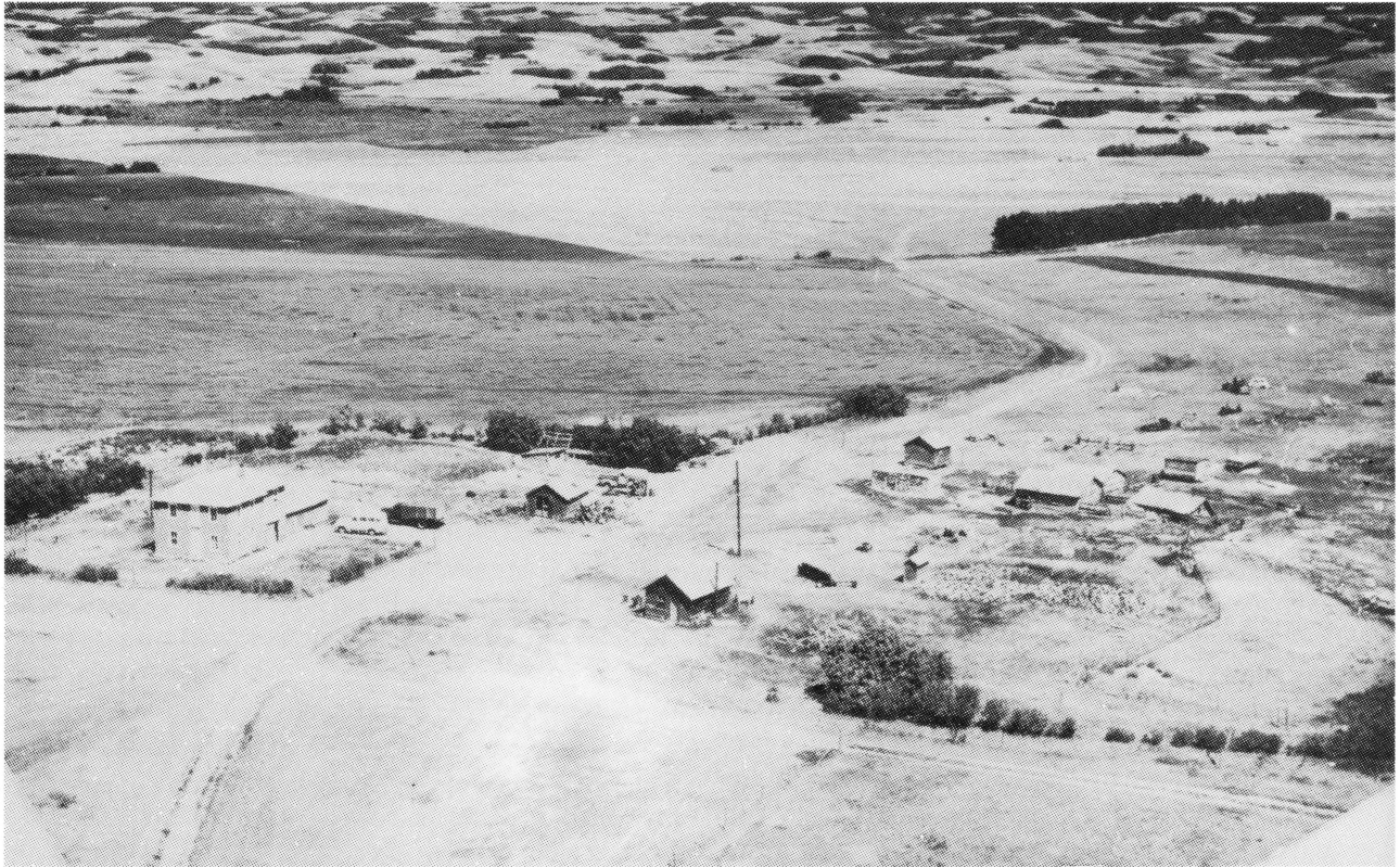
Aerial photo of ranch buildings
